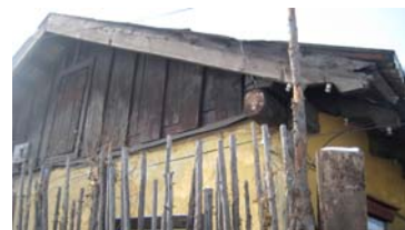
Fig. (4.1). Wood roof truss.
