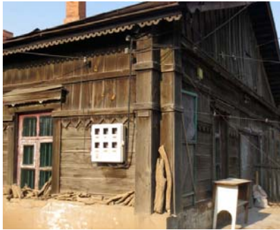
Fig. (2). Column in the corner of a wall (photographed by authors themselves).
