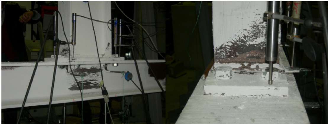
Fig. (10). a) Yielding of the panel zone b) Failure of the weld.
