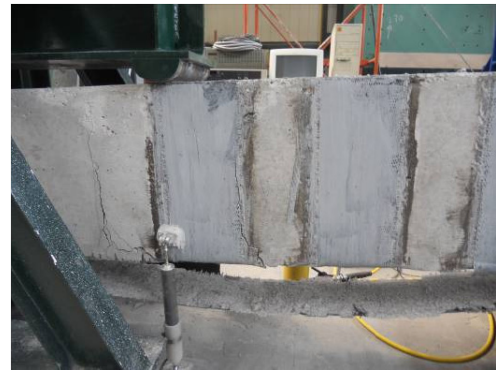
Fig. (9). Specimen 2 - Debonding of the CFRP strengthening system.
