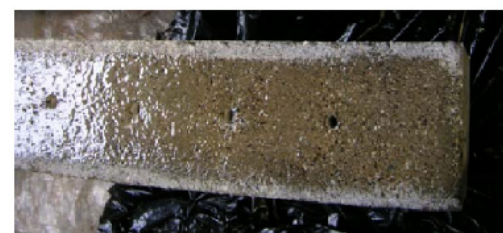
Fig. (4a). Drilling and placing of anchors.
