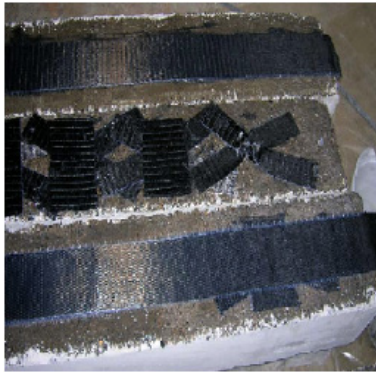
Fig. (4b). Placing of anchors and CFRP application.
