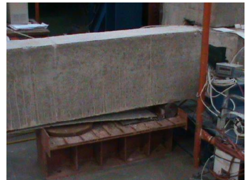
Fig. (13). Specimen 4- Debonding the CFRP sheets at the end of the test.
