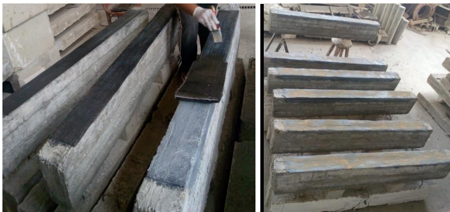
Fig. (4). Strengthened beam with CFRP.
