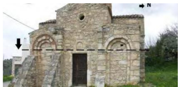
Fig. (2). An example of the effect of a combination of forces acted on a byzantine monument in Crete, of which the seismic load is the predominant force (Church of St. Demetrios near a village in the Rethymno district).
