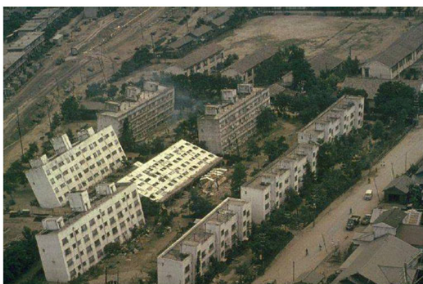
Fig. (6). Soil liquefaction June 16, 1964, Niigata, Japan, M_{max} 7.5. Photo: Joseph Penzien.
