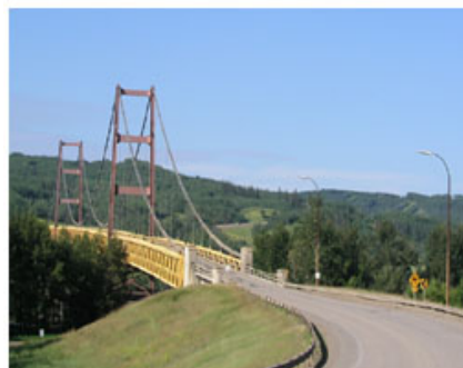
Fig. (16). A bridge over the Peace river (Canada, Alberta).
