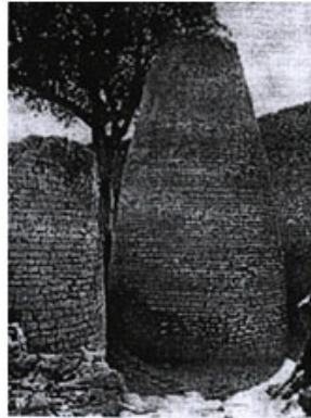
Fig. (10). A closed shell of an elliptic cross-section of the complex of Big Zimbabwe (Africa).
