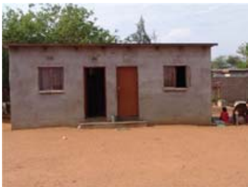
(a) SHHA Loan Improvement scheme house.
