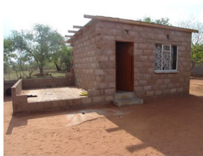
(b) One-room house built of concrete blocks.
