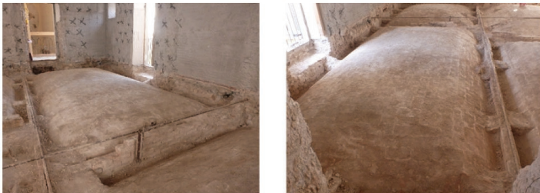
Fig. (2). Mansony pavillon vault during retrofitting works.
