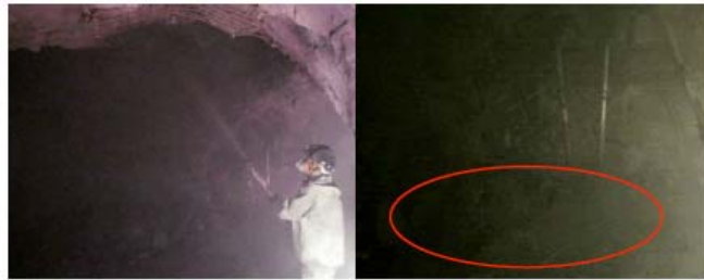
Fig. (8). Field test of metal net spraying concrete.
