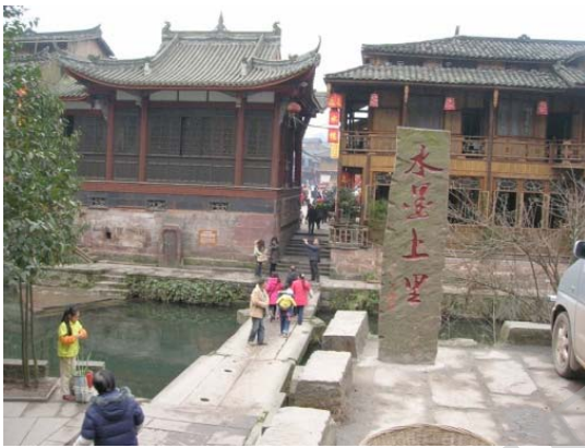
Fig. (13). Bridge that connects with the Opera Court.
