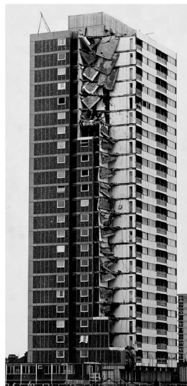
Fig. (1). The Ronan Point collapse.
