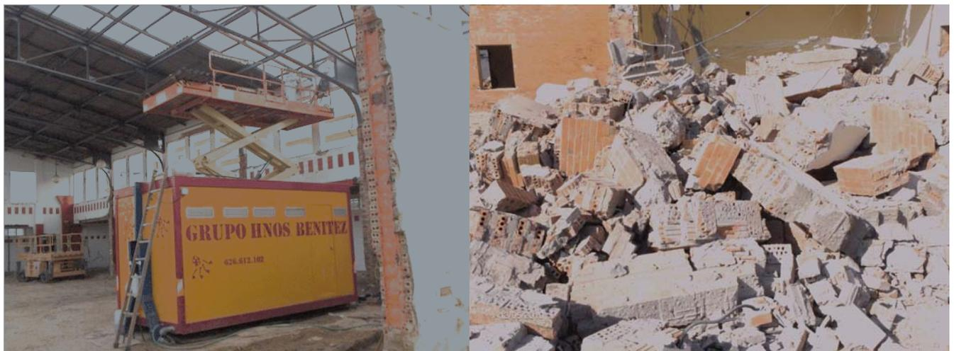
**Fig. (3).** In the picture on the left, panels containing asbestos are removed as hazardous material by an authorized manager, and on the right, bricks and concrete are treated as non-hazardous and are ready to be crushed and reused.
