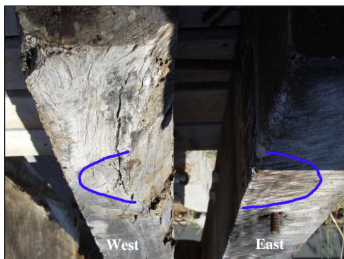
Fig. (14). Condition of the underside of the western half-cap on pier 1, pile 3.
