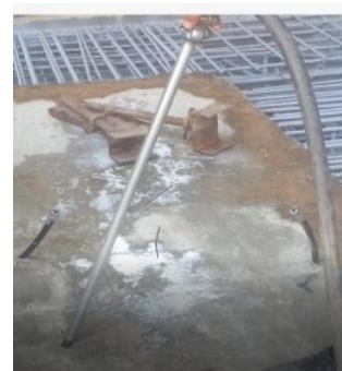
c) Applying pressure to move oil along duct
