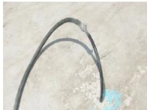
d) Connecting the grout injection to grout inlet
