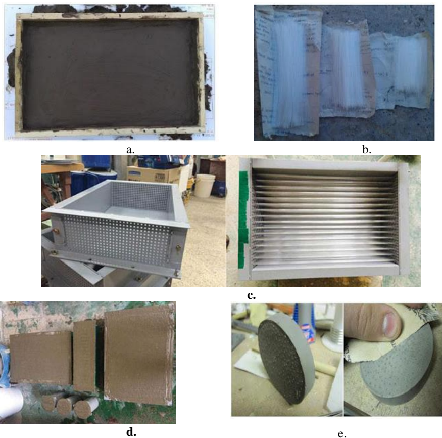
Fig. (6). Steps for the production of translucent concrete: (a). Preparation of panel; (b). Optical Fibers; (c). Fixing of fibers; (d). Concreting; (e). Cutting and polishing of the surface [52, 53].
