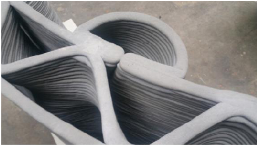
Fig. (8). 3D printed concrete structure (courtesy of Gosselin et al. [59])
