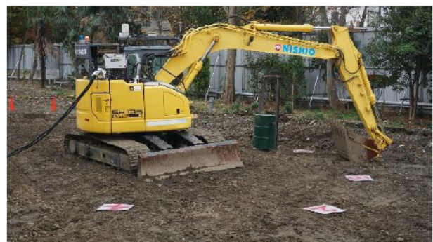
Fig. (6). Work site.
