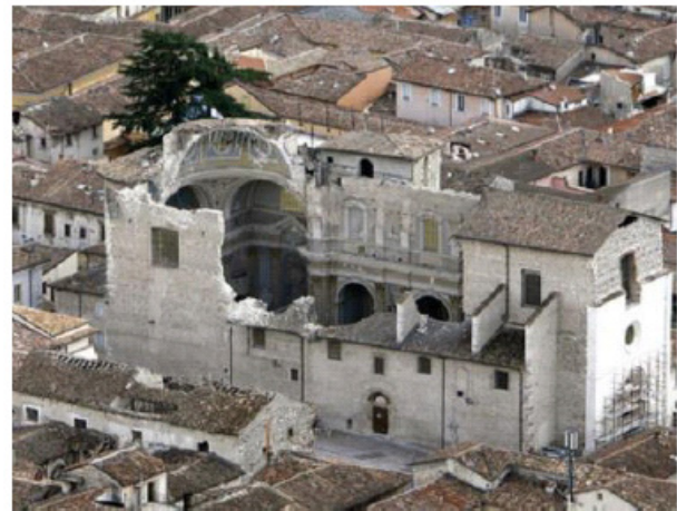
Fig. (3). Santa Maria church in Paganica (Italy) after the earthquake of 2009.
