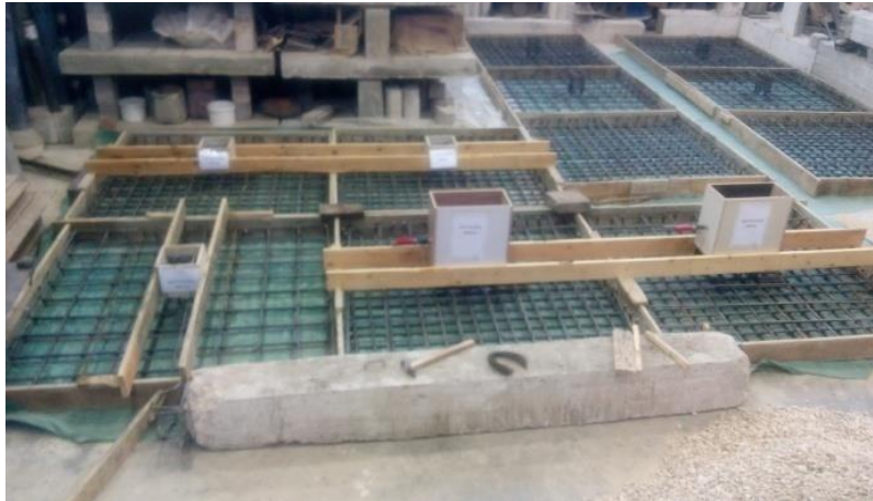
Fig. (3). Wood forms and RFT meshes.
