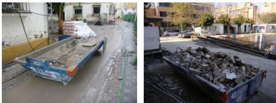
Fig. (7). Skips for waste removal.
