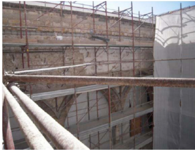
Fig. (11). Consolidation of irregular masonry walls of loggia.
