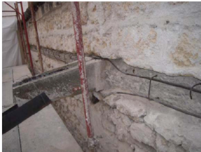
Fig. (12). Consolidation works on reinforced concrete curbs.
