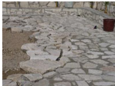
Fig. (4). Construction of pavement from calcareous chalks [3].
