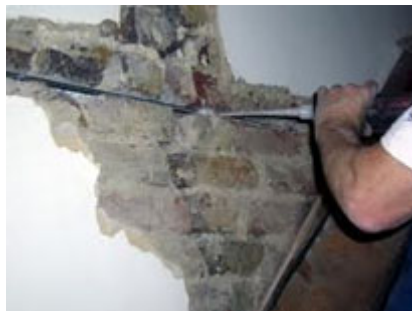
Fig. (12). Crack widening by removing the mortar, loose stones and gallets [3].
