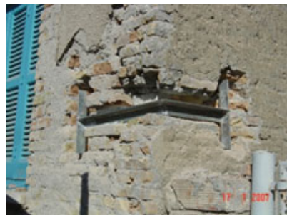
Fig. (13). Reinforcing of the corner by galvanized metal element [3].
