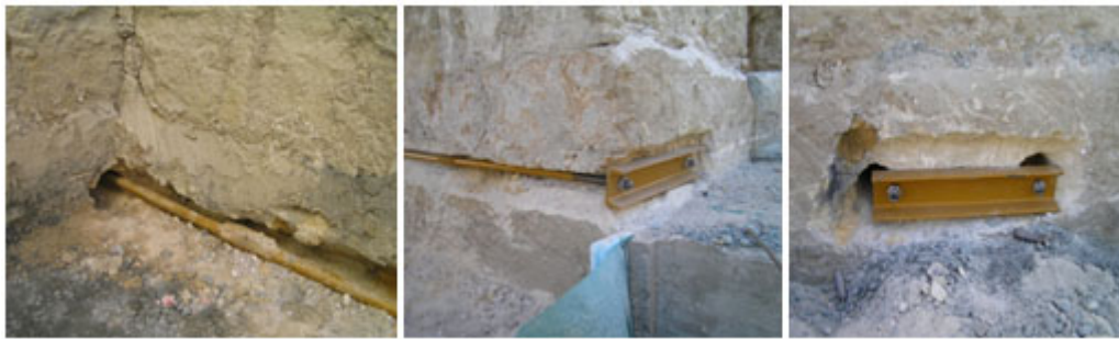
Fig. (16). Tendons installed to masonry wall [3].
